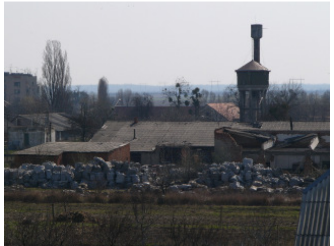
Chaotically dumped big bags with a hazardous substance Premix in Zakarpatya oblast (2005)
